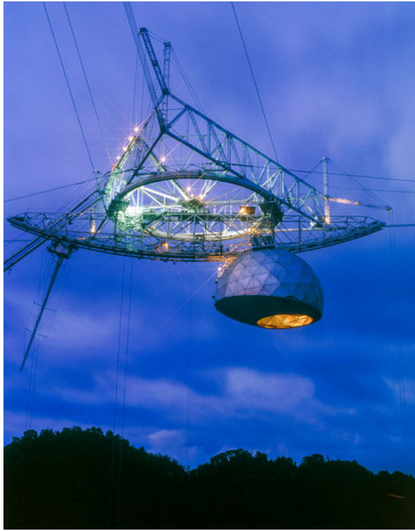
The 110-ton Gregorian dome, added to Arecibo in 1997, boosted capabilities but the added weight may have hastened the platform's collapse. DAVID PARKER/SCIENCE SOURCE
